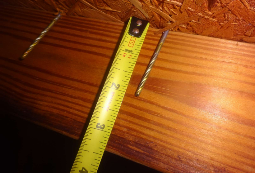
8d nails verified
